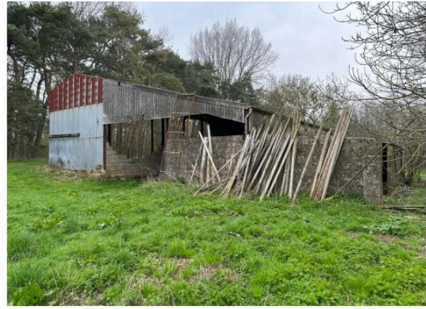
2. South west facade of existing barn
