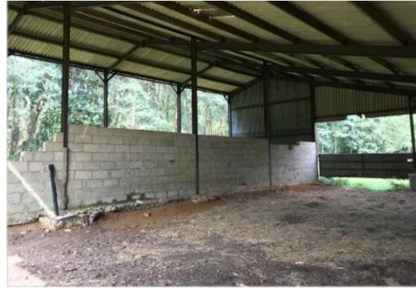
8. Interior of existing barn
