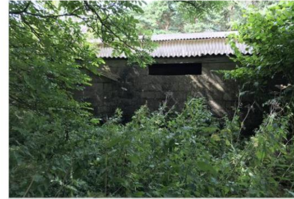
9. Existing lean-to to south of the barn
