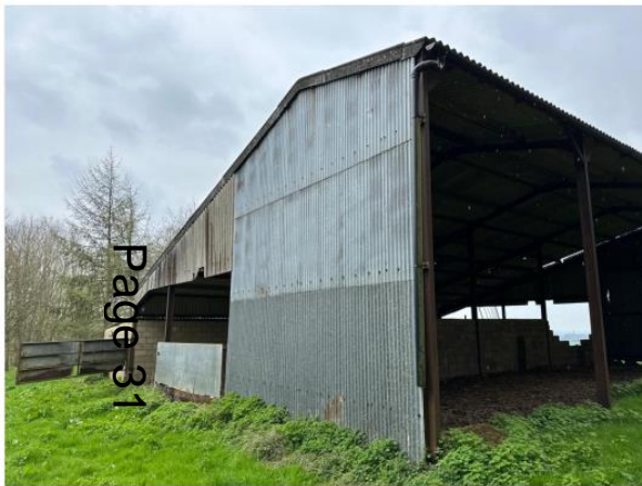
10. Existing barn is clad in a mixture of galvanised steel and asbestos
