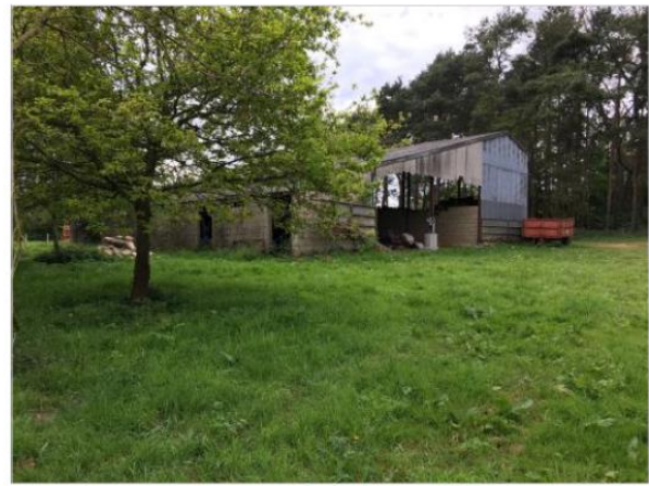
5. Existing barn from the east
